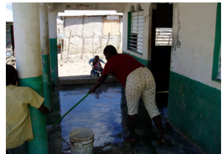
Below - pictures of the concreted floors
